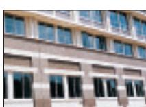
Precast thin brick panels eliminate the need for lintels, sills, weep holes and tie rods.
