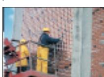
After the panels are tilted and erected, the snap carriers are removed.
