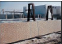
Brick precast panel ready to be cleaned. Panel is cleaned to remove concrete leakage.
