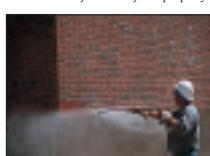
Brick panels are cleaned with hot, high-pressure water.
