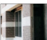
Erected panel shows thickness of concrete bonded to thin brick.
