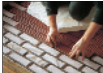
Brick are placed over retarder paper in gasket liner
