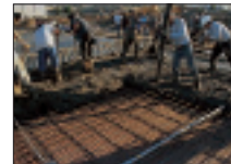
Concrete is poured and vibrated to insure mortar joints are filled properly.
