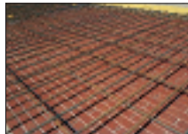
Rebar is placed and panel is ready for concrete.
