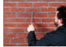
When mortar is thumb-print hard joints may be tooled.
