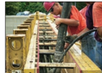
Vertical forms are set with rebar and concrete is poured.
