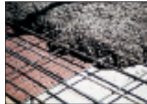
After steel reinforcing is in place, concrete is poured over the assembly.
