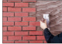
Mortar is applied with a 1/4" notched trowel.
