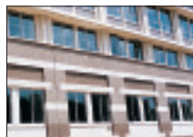
Precast thin brick panels eliminate the need for lintels, sills, weep holes and tie rods.
