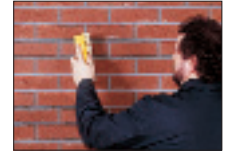
Brush joints to remove excess mortar before mortar cures.
