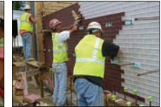
Thin brick is pressed into the pockets of the Rim Snap system face down.
