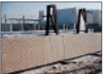
Brick precast panel ready to be cleaned.
