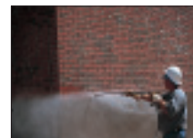
Brick panels are cleaned with hot, high-pressure water.
