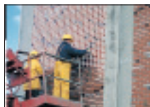
After the panels are tilted and erected, the snap carriers are removed.
