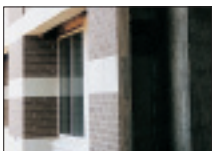
Erected panel shows thickness of concrete bonded to thin brick.
